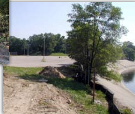
Under construction near Atwood Stadium
